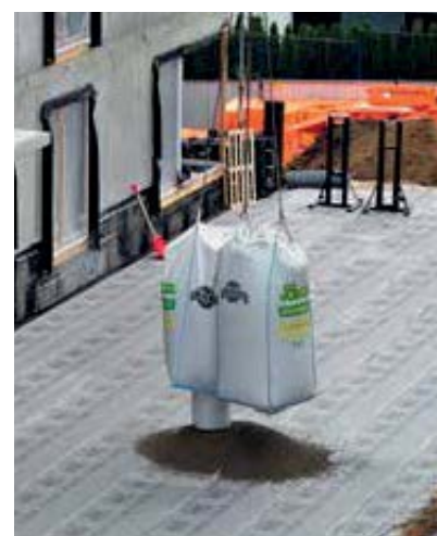
The material was fed directly to the site of its placement
